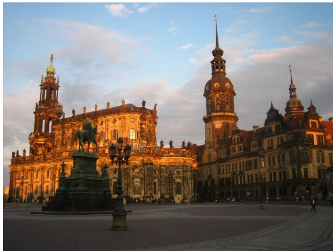
Slika 2: Historical Part of the City of Dresden
